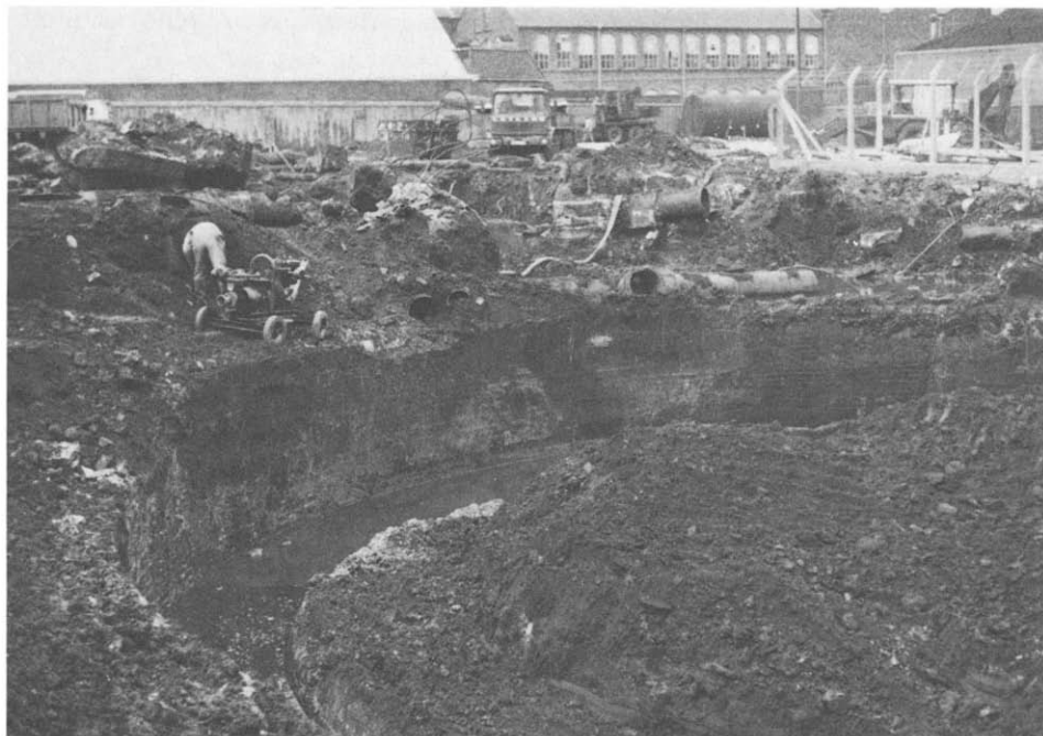
Fig 2 Excavated gas holders
